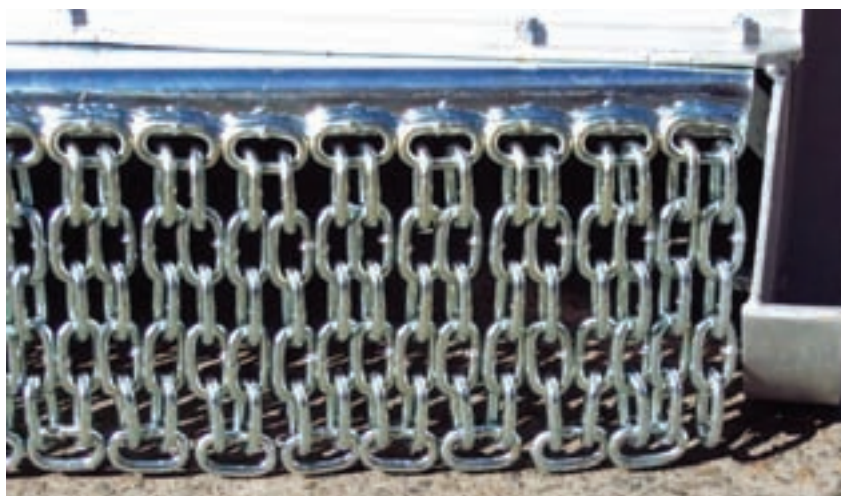
Figure 3: Chain curtain, using continuous chain, looped (top and bottom) and fixed to the supporting structure by welding. Alternative methods of securing chain, such as slots and retaining rod or wire, are also suitable.
